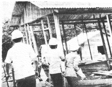
The demolition squad
